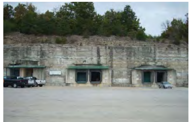
The Mountain Data Center
