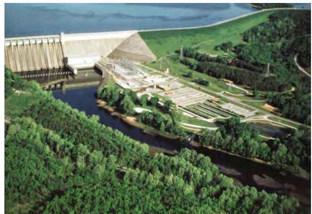
Aerial view of Table Rock Dam
