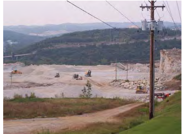
Tanstone development under construction
