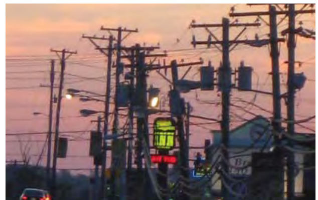
Overhead utility poles along 76 Country Blvd.
