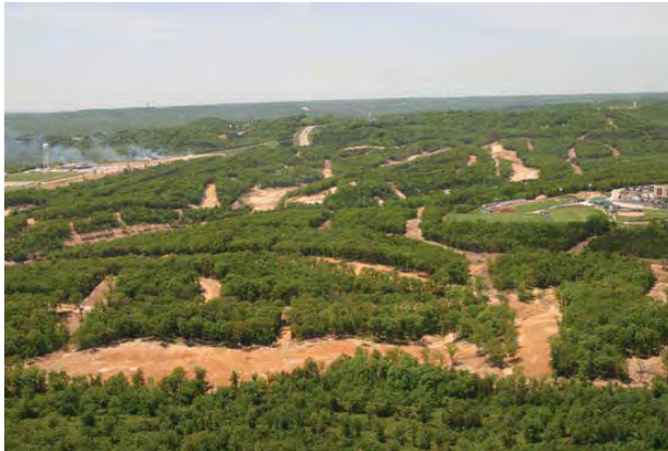
Branson Hills and Payne Stewart Golf Club under construction
